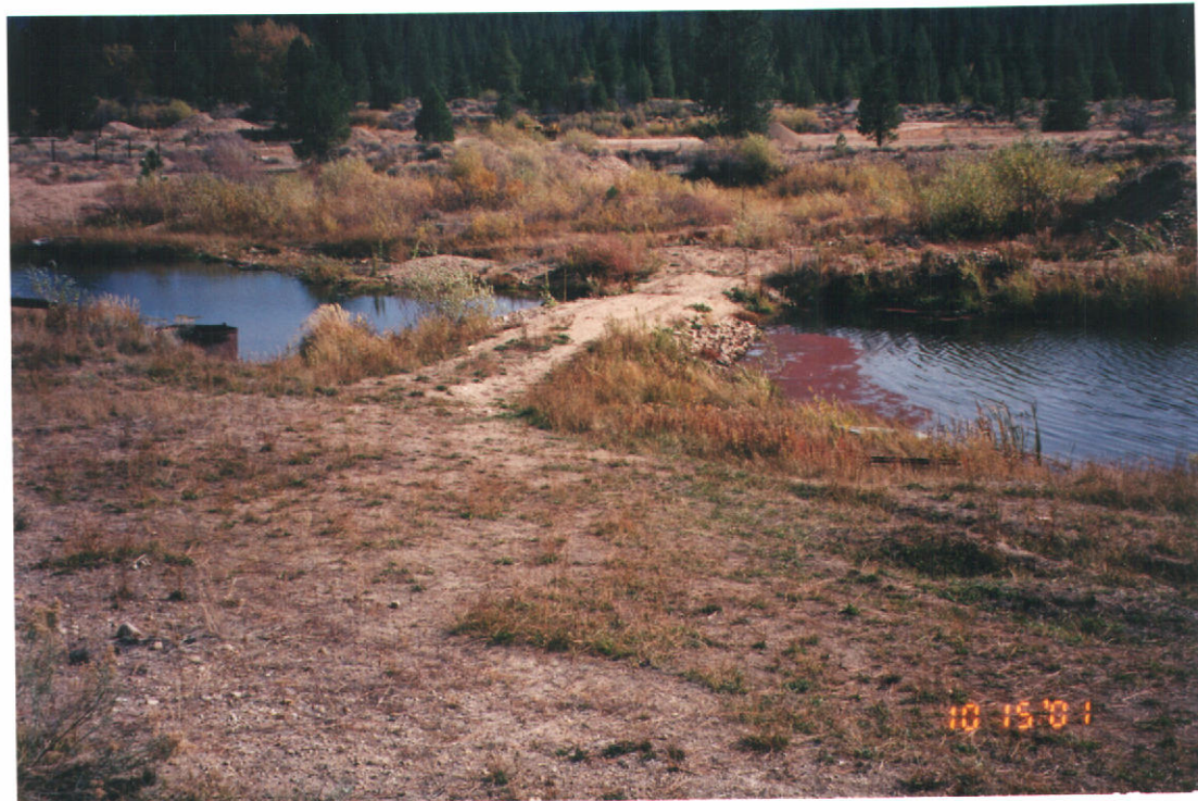
PHOTO # 3 DIKE USED TO REGULATE THE FLOW BETWEEN THE PONDS IN THE NESW & NWE, S6
