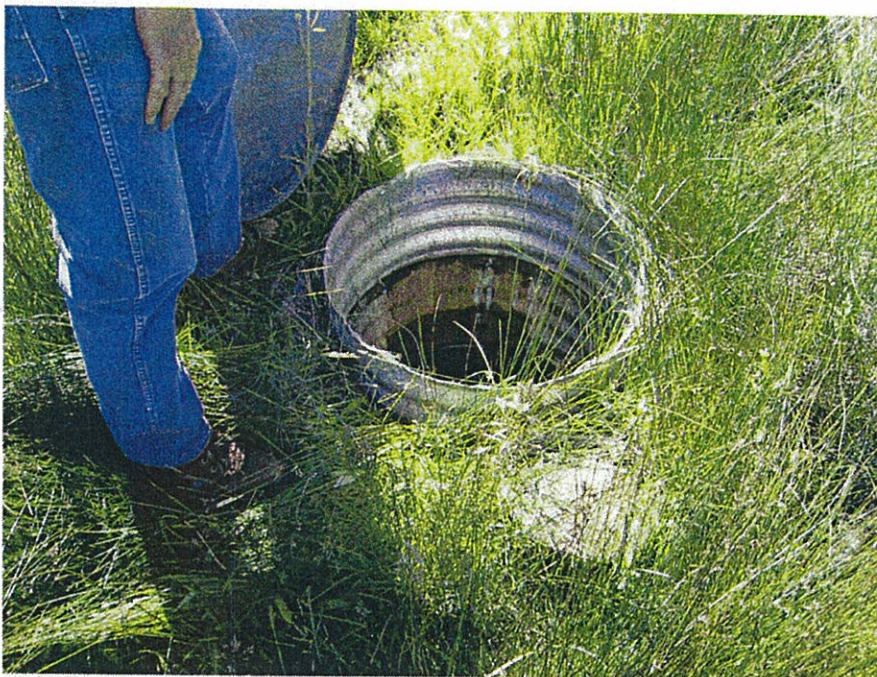
Catch basin located to west of boggy area.
