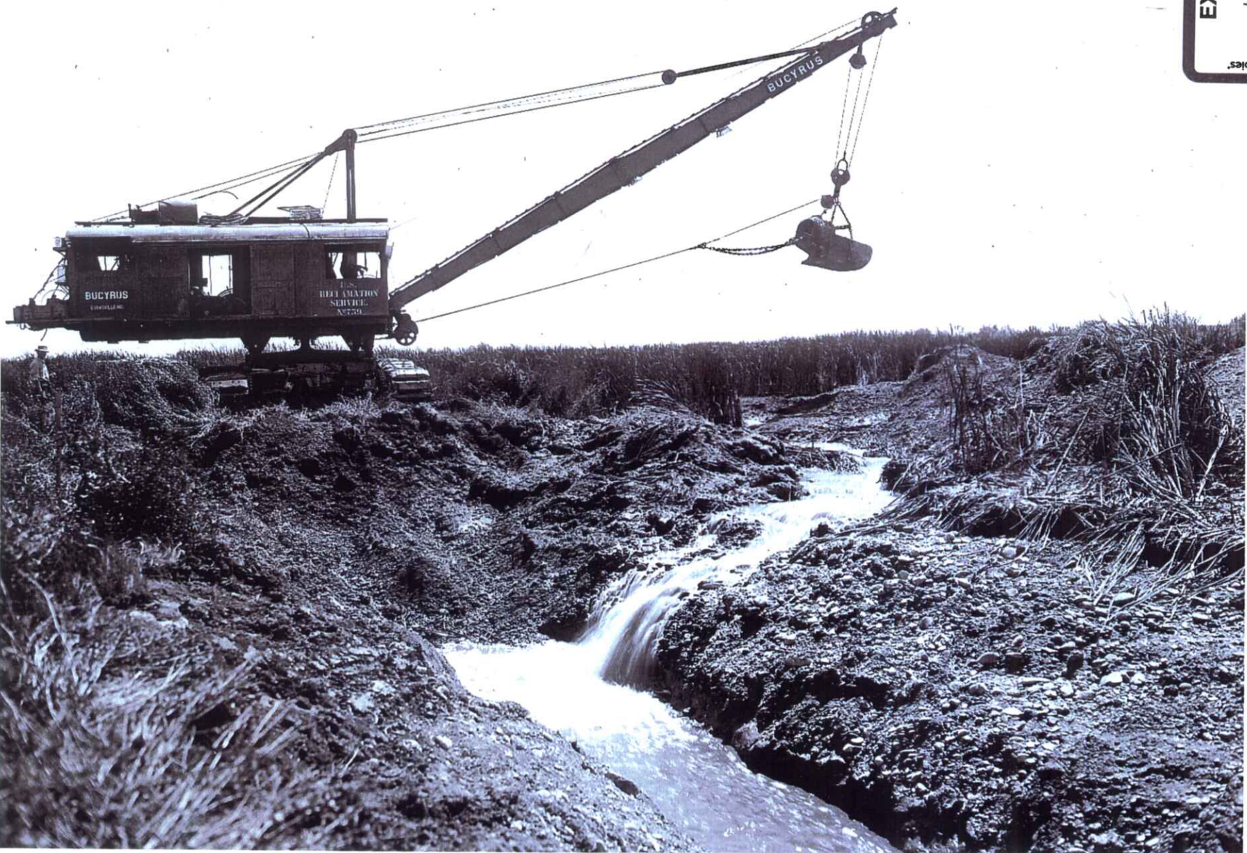
P4-100-3348 Electric dredge excavating Purdam Slough Drain on Lemp's ranch. Arrowrock Division, Boise Project, ID. USBR photo by Walt Lubken. Jun 22, 1914.
