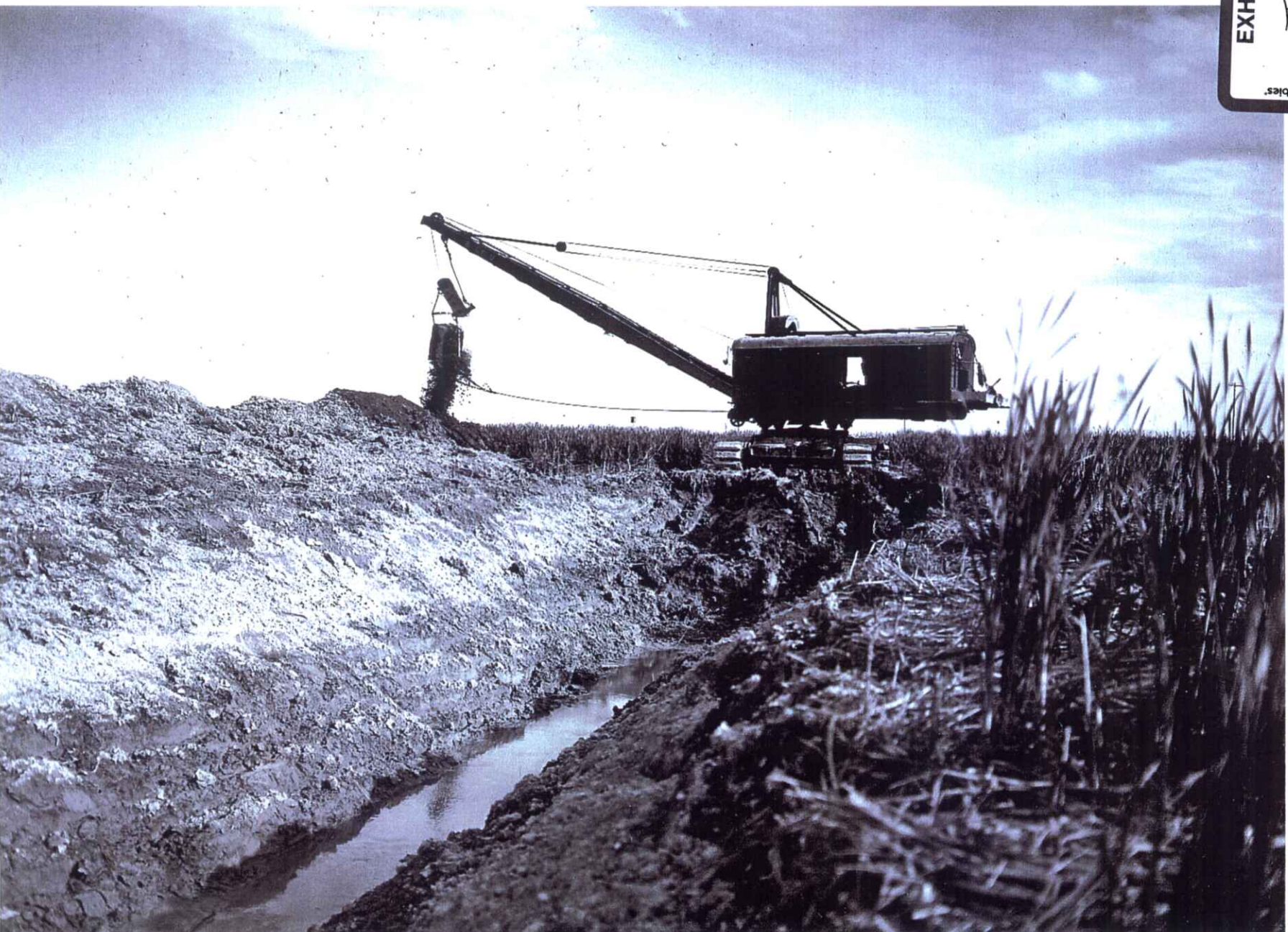
P4-100-3347 Electric dredge excavating Purdam Slough Drain on Lemp's ranch. Arrowrock Division, Boise Project, ID. USBR photo by Walt Lubken. Jun 22, 1914.
