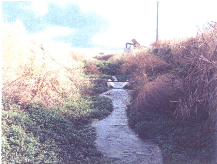
Photograph 1: Water Right No. 63-27475 point of diversion from Purdam Gulch Creek in background with Trapezoidal Flume in mid-photo.
