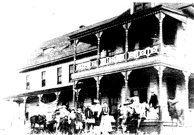
At the old Algenia Ranch house. (courtesy of Ken Wright)
