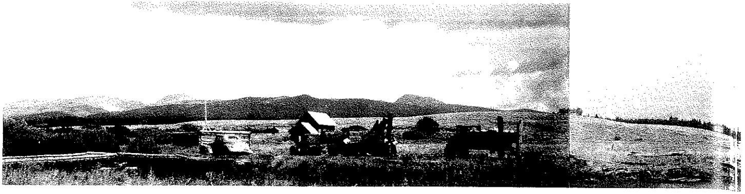
Trude/Wilkins Ranch buildings being trucked across the river before the reservoir waters come! The truck broke down in the middle of the river so the truck on the bank is pulling it to shore. Looking upstream, the building in the distance is the Guest House, now known as Lakeside Lodge, -- Picture taken in 1935. (courtesy of Hal Wilkins)
