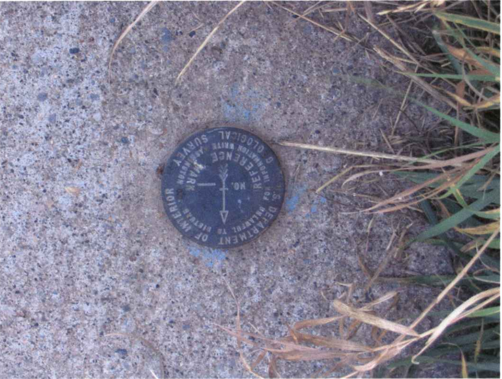
A22-12528 & A22-634; Survey marker on pump pad
