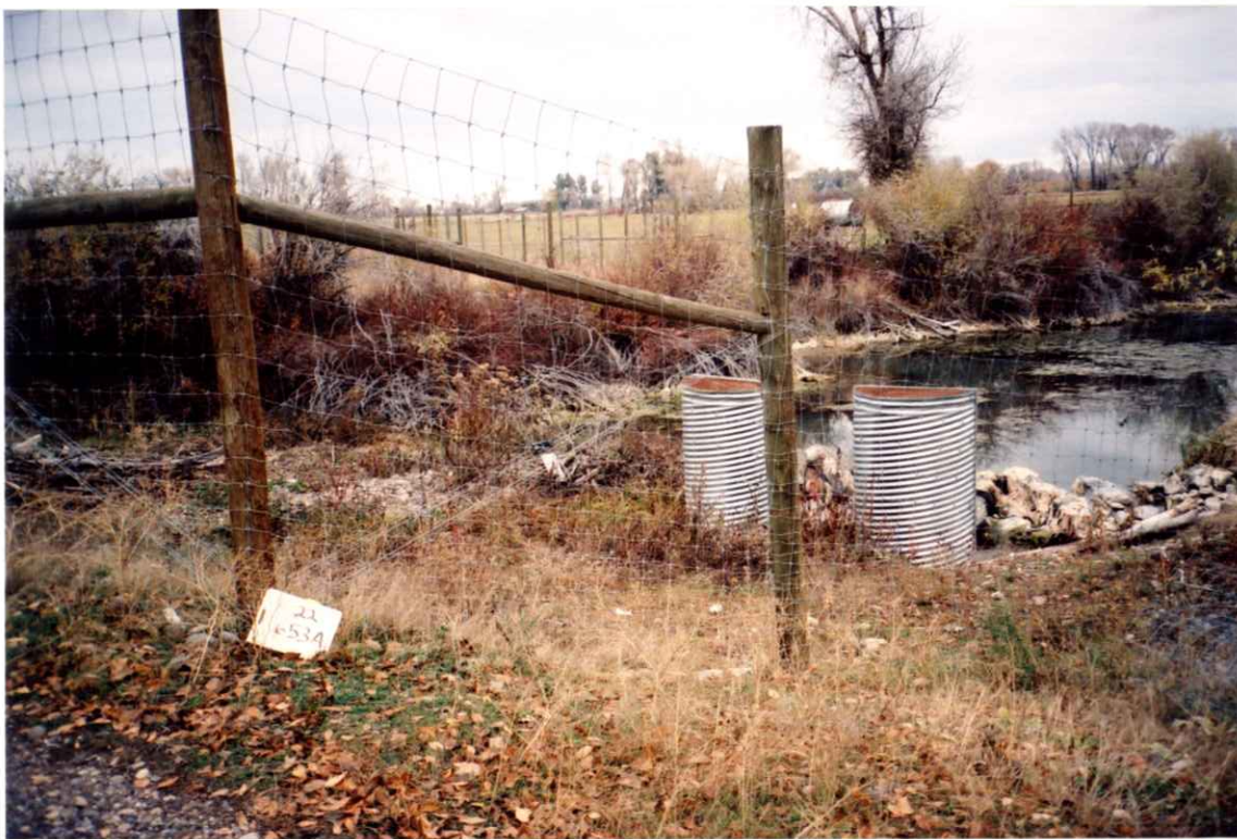
A22-653A end of slough where return culverts carry excess water to Snake River photo # 3 on map
