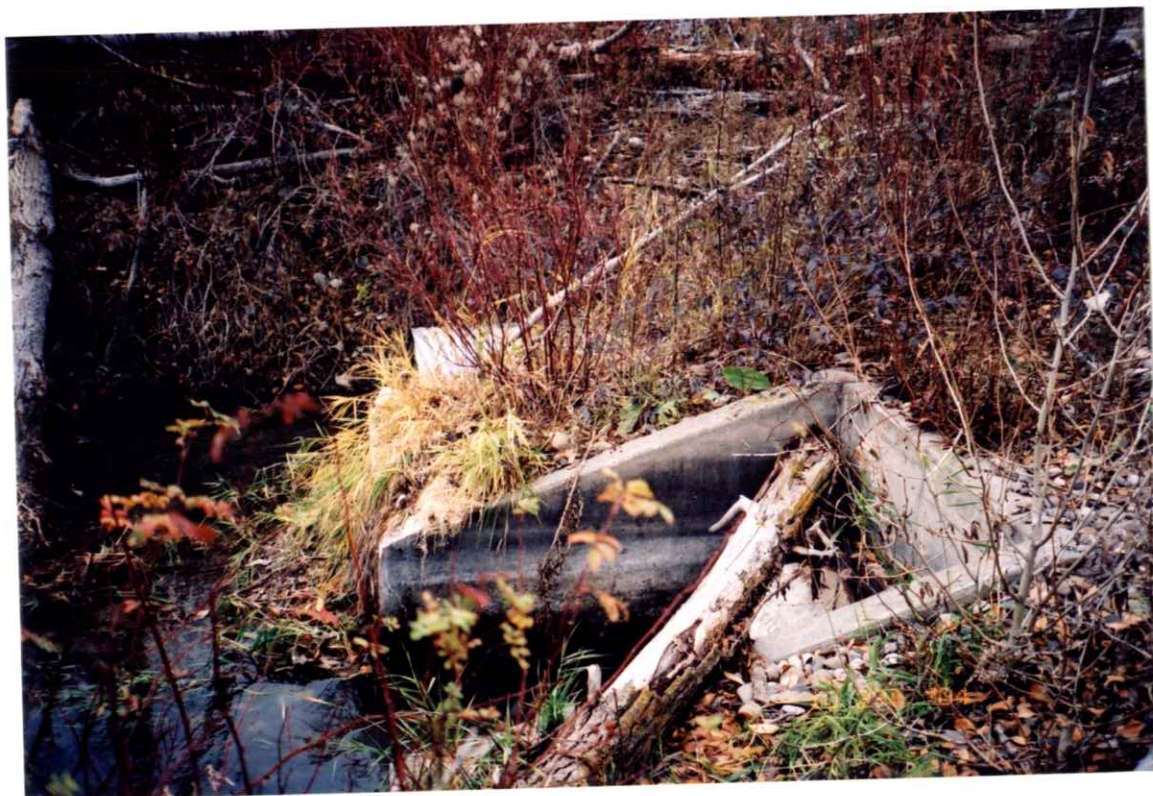
A22-653A flapper gate @ discharge end of return culvert.
