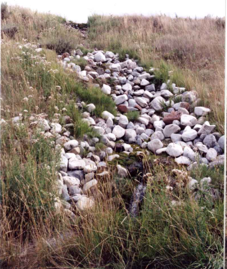
② Drop structure at laypoint 23 looking SE 9 Sept 05 Bac
