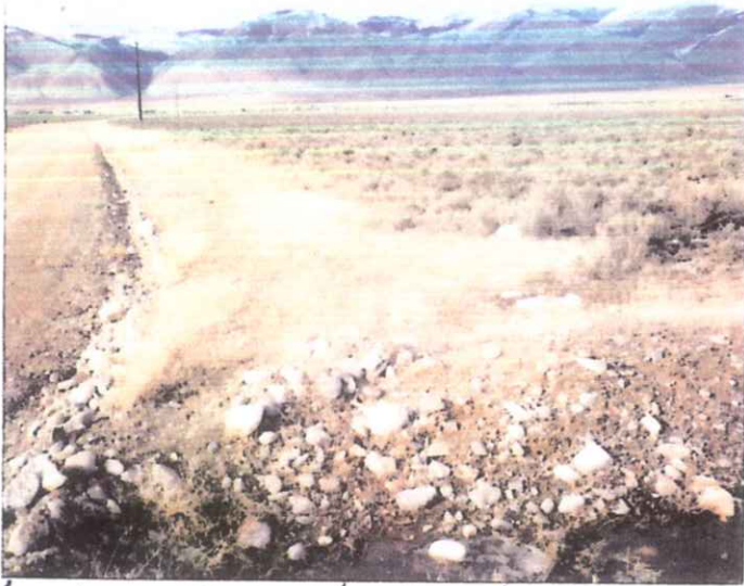
Looking towards headone, POU on right hand side of Adams Road 3/16/07
