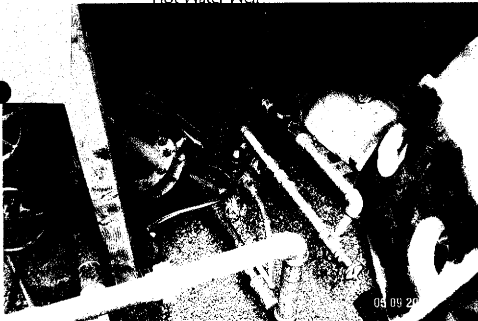
Associated Plumbing with Hot Water Well
