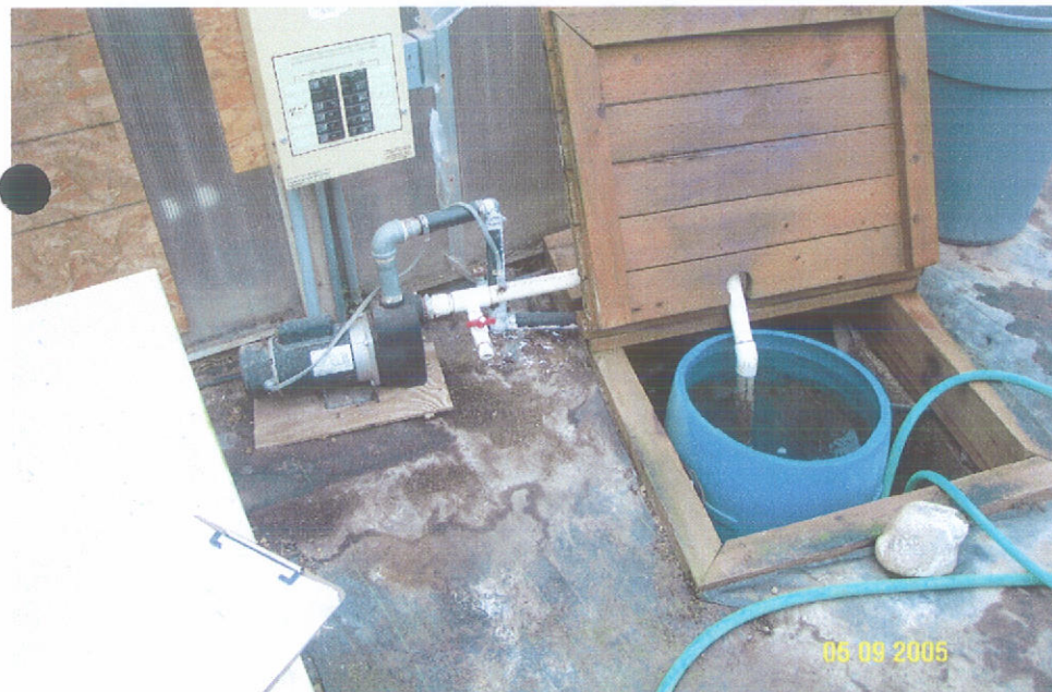
Hot water recycle—Booster pump for heating
