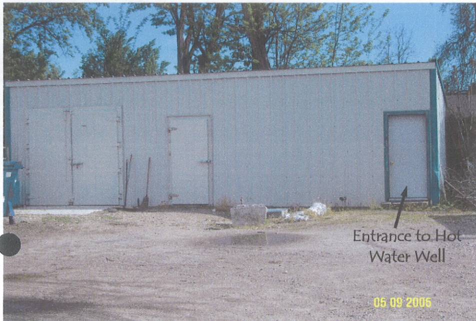
Hot Water Well head building
