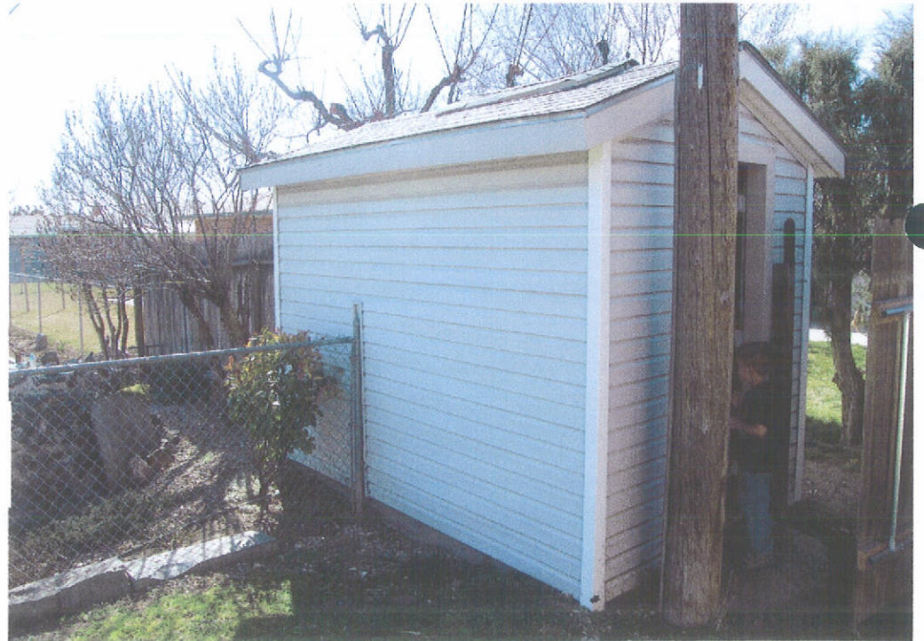
Pump House Looking Southwest
