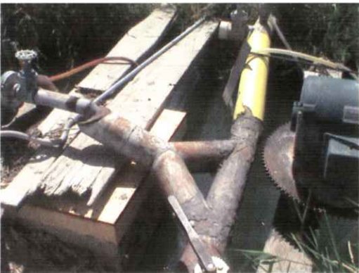
Point at which water from river ties in with water from BID.
