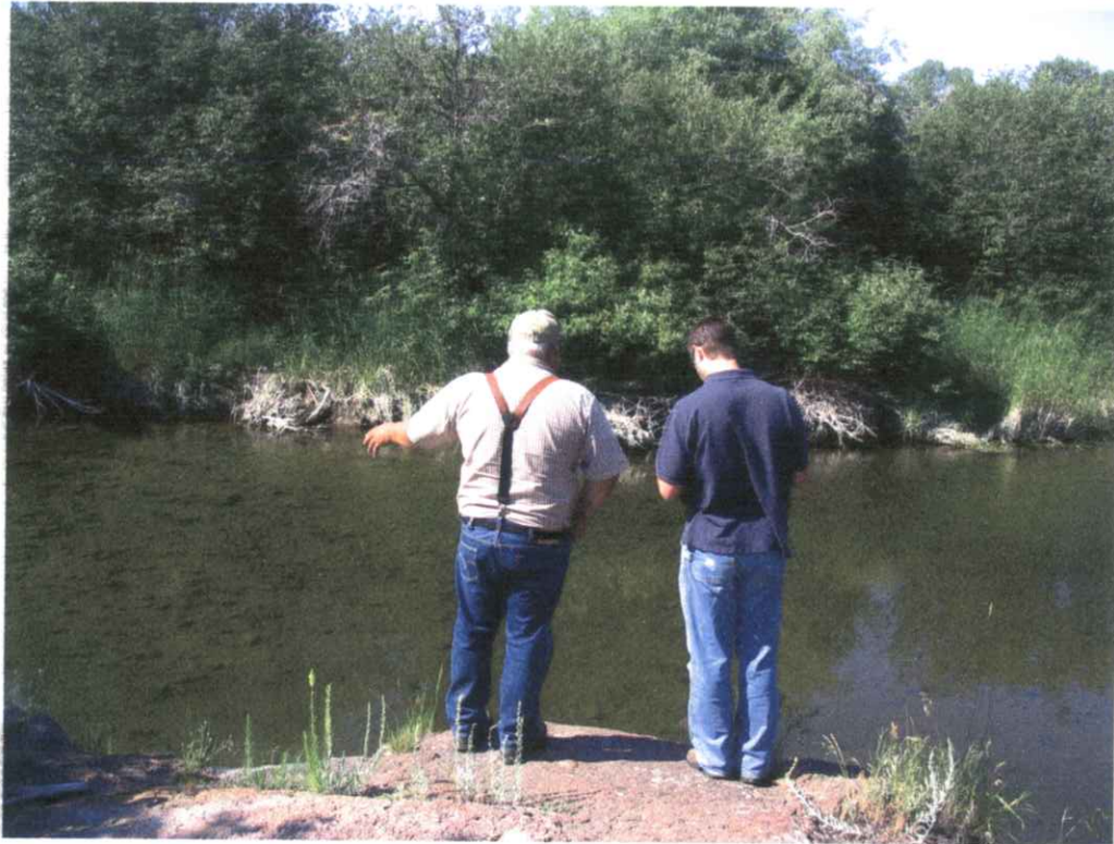
Spring / wastewater return area & pump location
