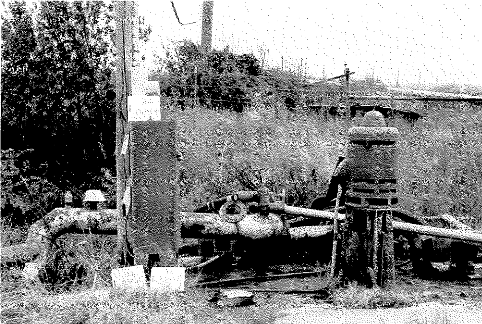
Photo #1, POD looking south east.
