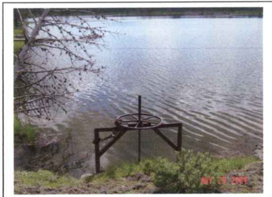
Point of Diversion: North side of dam. T11N, R43E, S06, NWNE. Photos by: RDH
