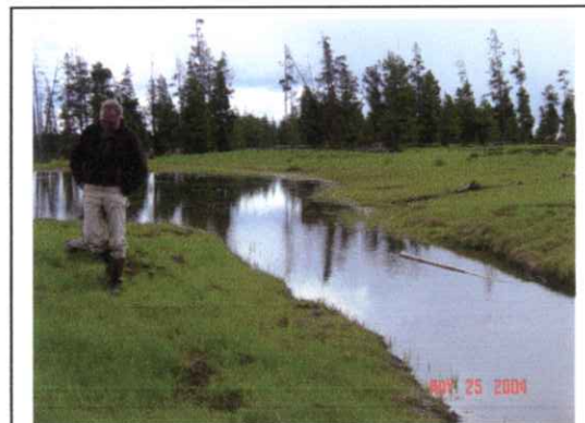
Spillway: On South side of dam.
