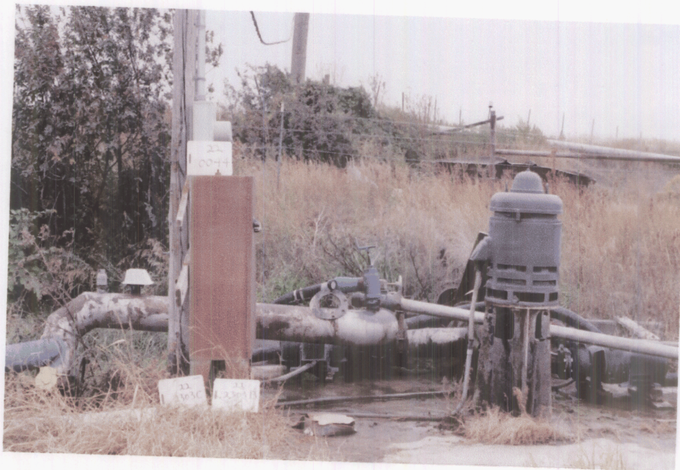
Photo #1, POD looking south east.
