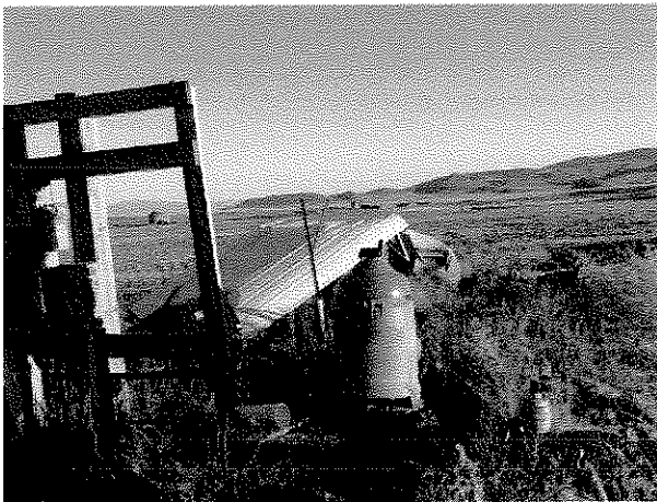
Photo 2. Point of diversion-looking southeasterly.
