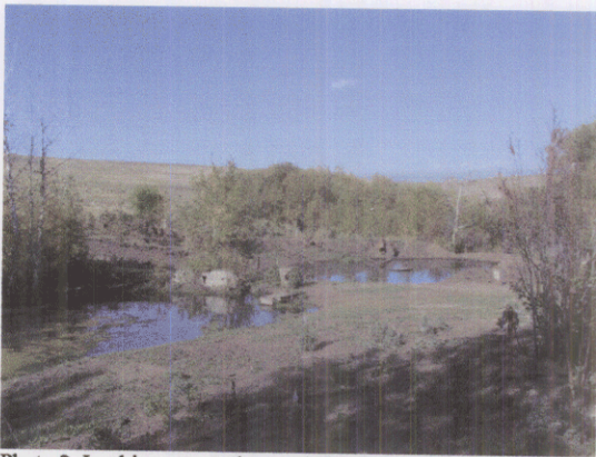
Photo 2. Looking east at the ponds for the gravity system.
