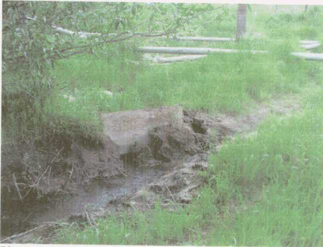
Photo 1. Diversion on Joe Willey Creek.
