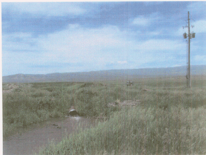
Photo 5. Looking Northeasterly at canal and pump.
