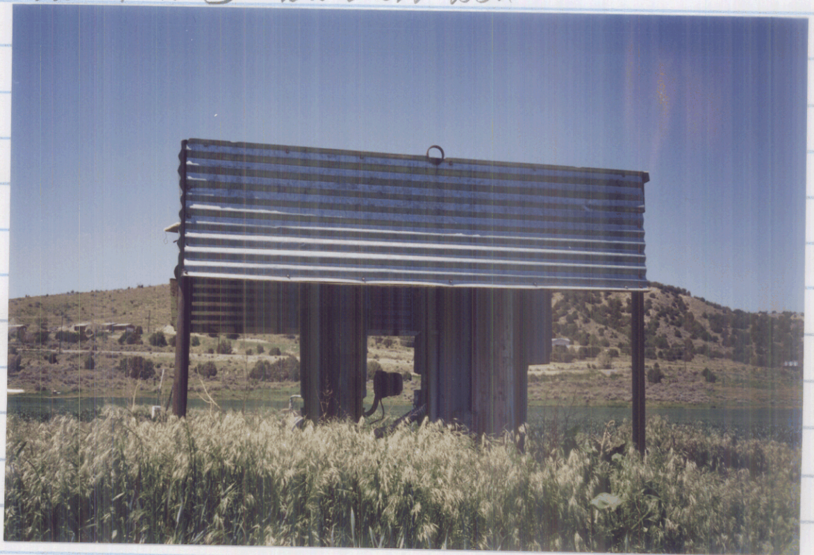
Looking SE @ NW most well
