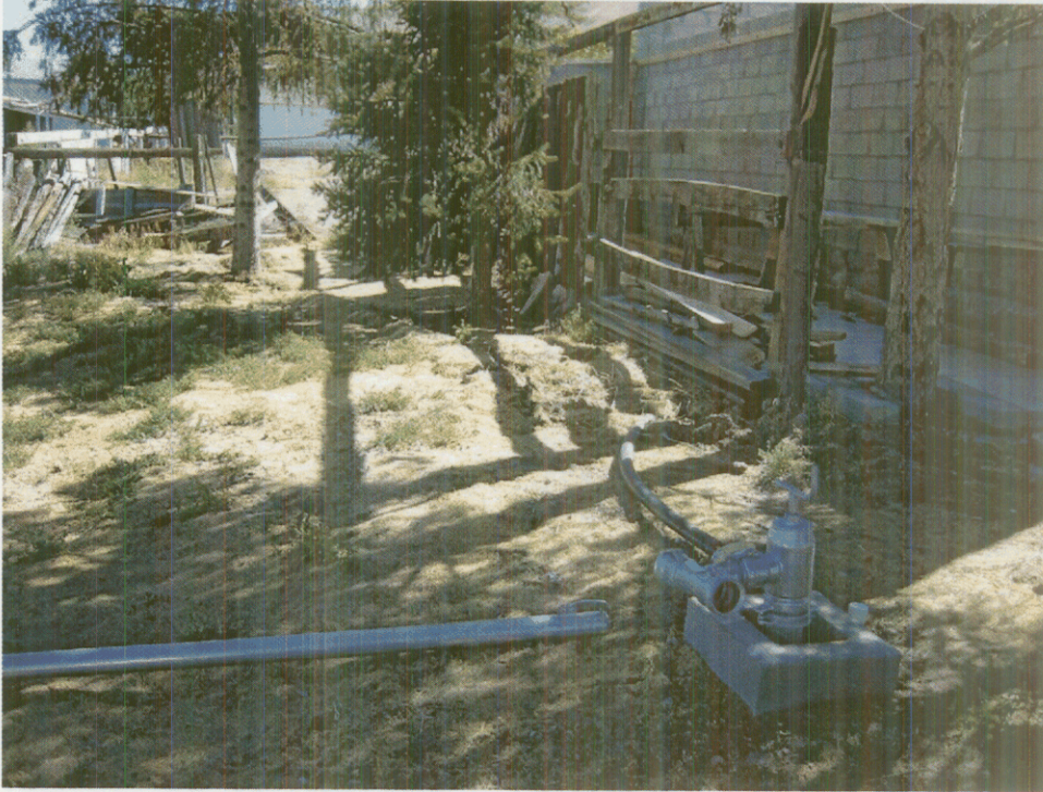
Looking North at new irrigation system put in place to replace old system (csaxton).
