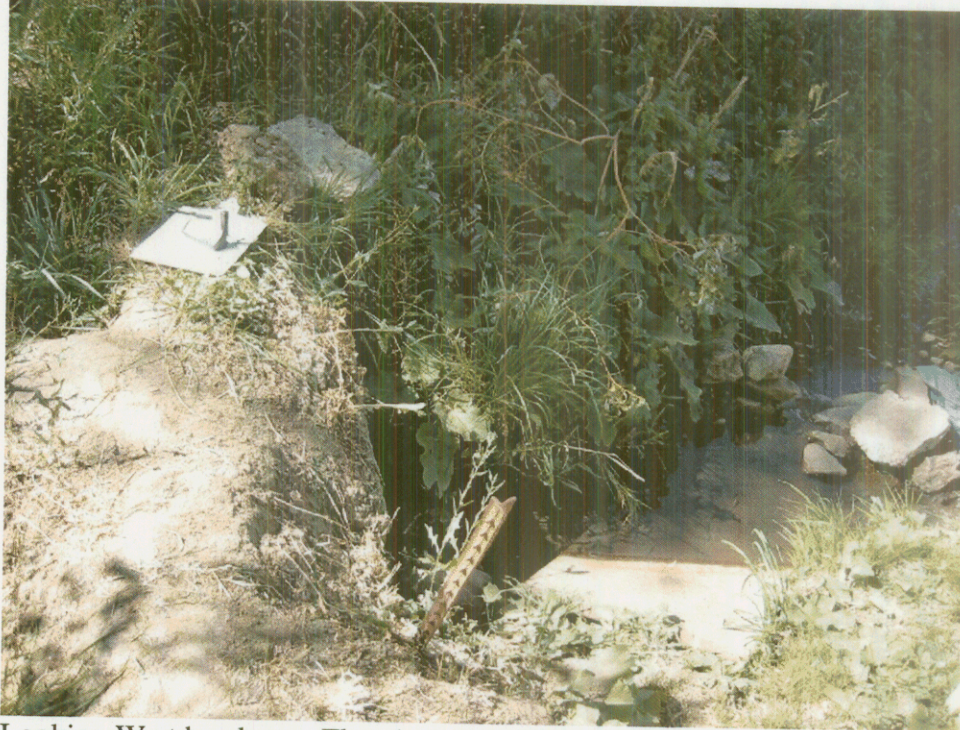
Looking W at headgate. Flow is to the right of the picture (csaxton)
