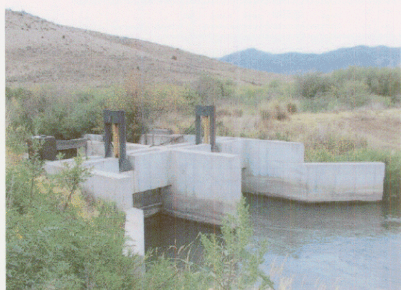
Photo 7. Head of the canal system.
