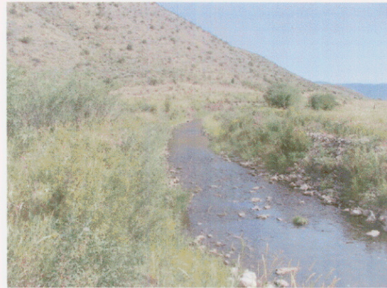
Photo 2. Feeder Canal at Toponce Creek.
