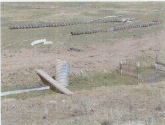
Photo 7. Looking north at southwest corner of the second pond.
