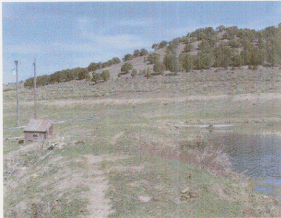
Photo 5. Looking north at 15 hp pump to the risers.
