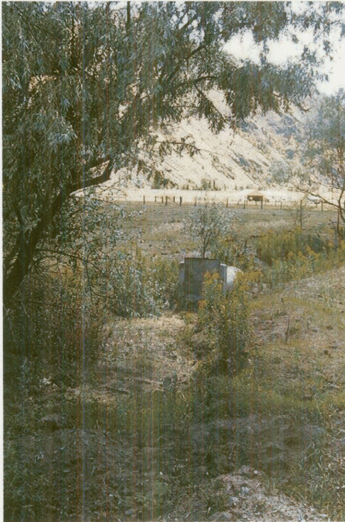
Looking SouthWest. Old concrete diversion (csaxton 10/31/01).
