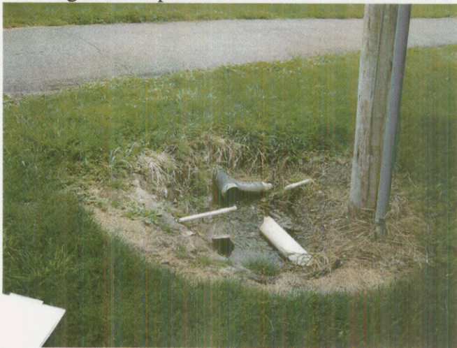
Looking NE at where water enters claimants property through the piping delivery system (csaxton).
