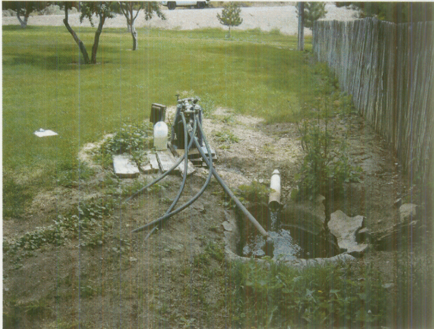
Looking North. Pump to divert water from cement catch basin.
