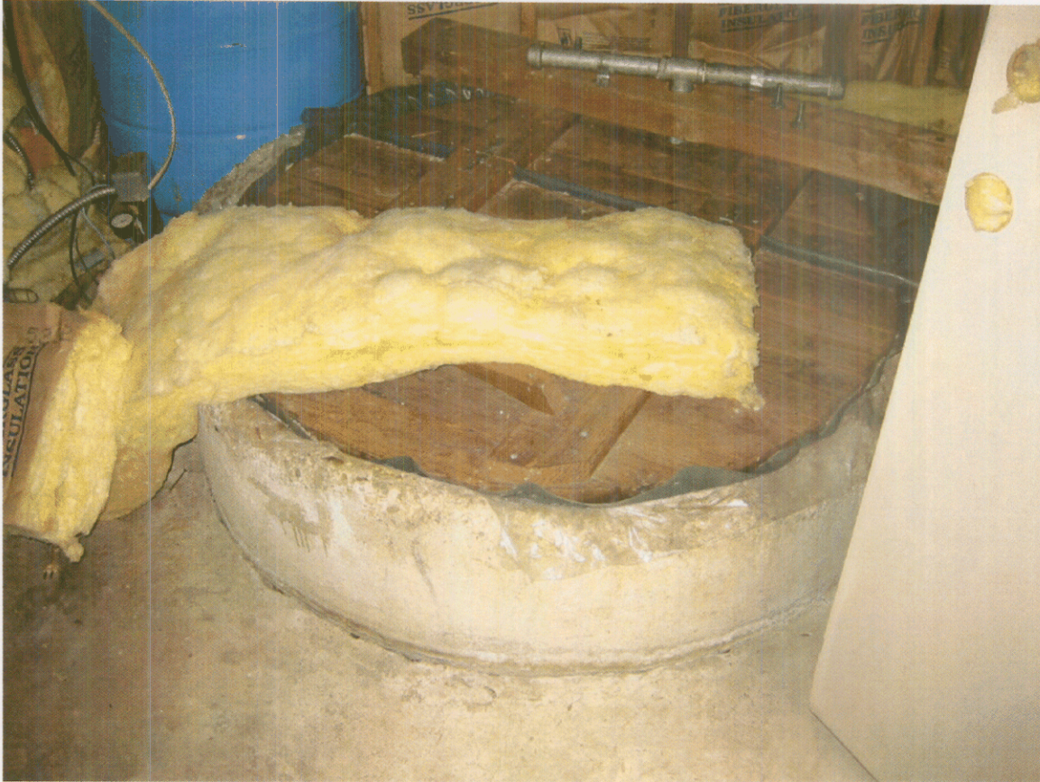
Looking inside of the spring house. Picture shows the catch basin that captures the water (csaxton 8/8/02).
