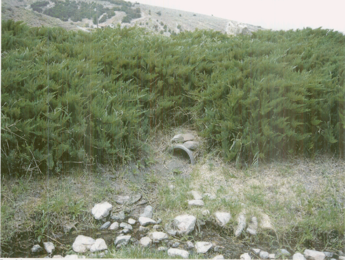
Looking West at historical culvert that conveyed water to West side of driveway to claimed POU. Now sprinklers are used (csaxton 8/8/02).
