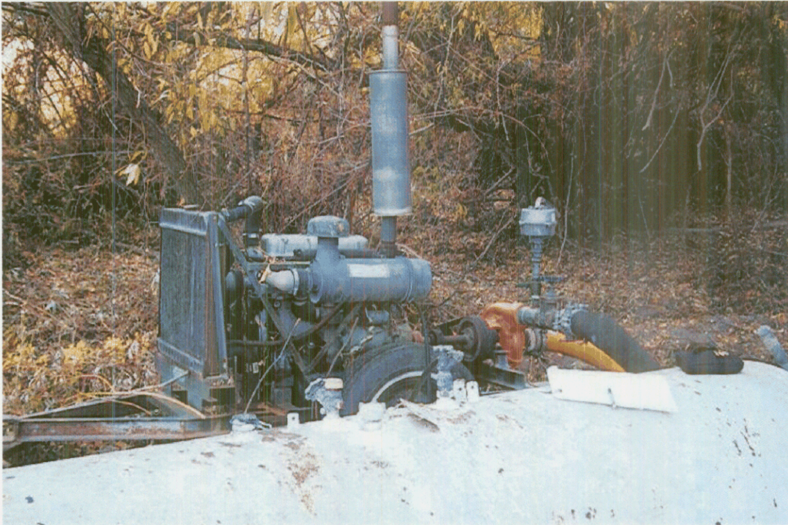
Looking west. Mobil Diesel powered pump. HP – Unknown: Model – VRG155: Size 3/ 8x3 ¾. White tank is the fuel tank. Pocatello creek to the right of the picture (csaxton 10/25/01).
