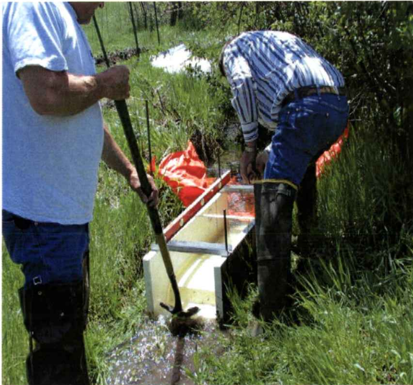
Steve Hebdon and Al Ruberry installing the 15" broad crested weir-flume on West Creek.
