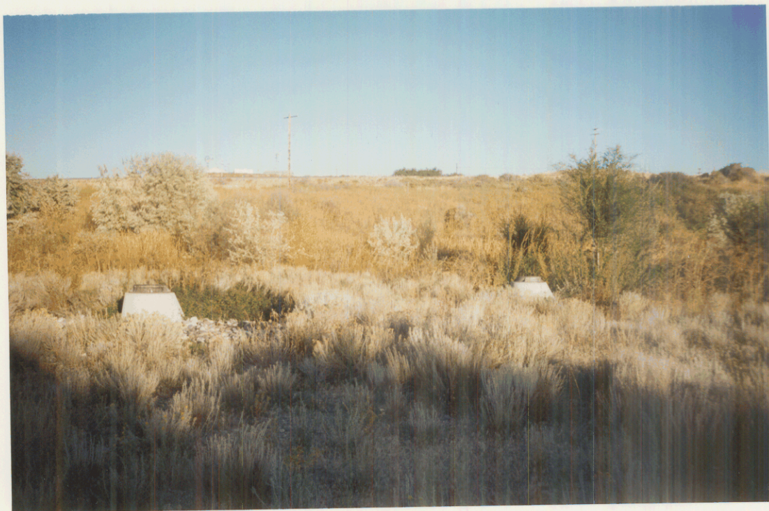
* PHOTO SHOWS DIVERSION AREA
