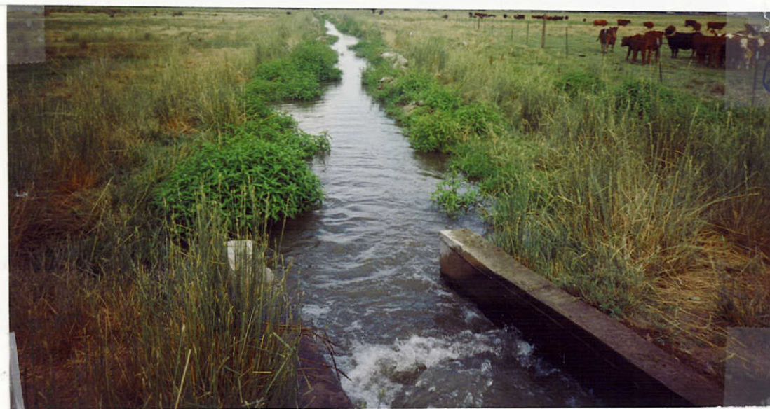
② Cement box in NWNW T05S R03E S. 5 to along south edge. Looking North along ditch. Water can also be Released into field w/ cattle
