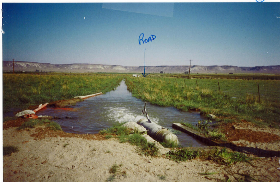
② Outlet on middle ditch. Looking NORTH 08/24/1994
