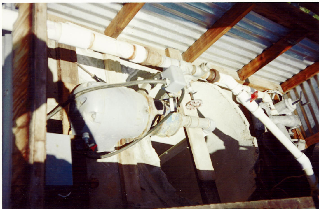
Photo #1-7 Looking into the Pump house showing The Pump and Corrugated Well Casing.
