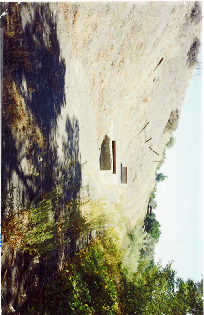
Access ports to infiltration gallery.
