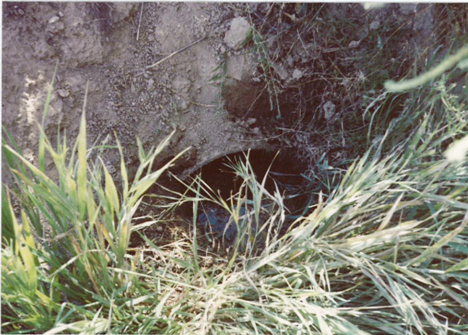
Photo #2 This 8" culvert carries the waste water under the road.
