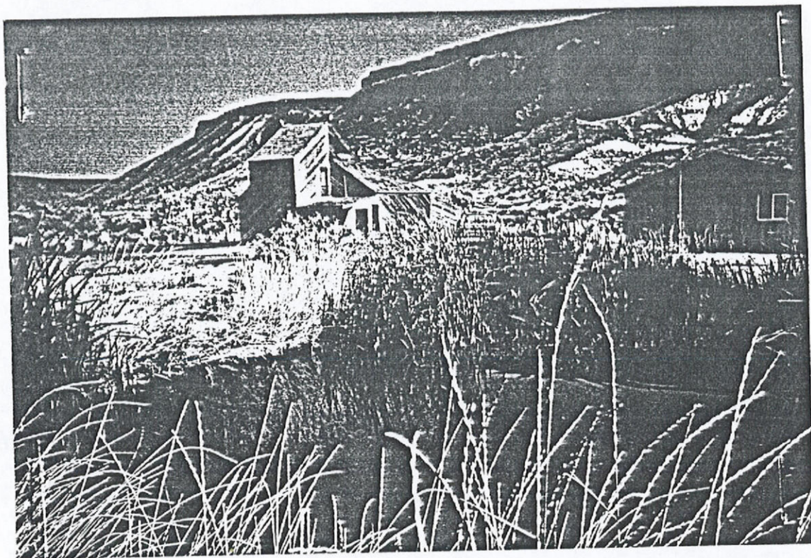
P.D. & P.U. the well is located in the garage visible on the right side of the photo. Looking North- northwest
