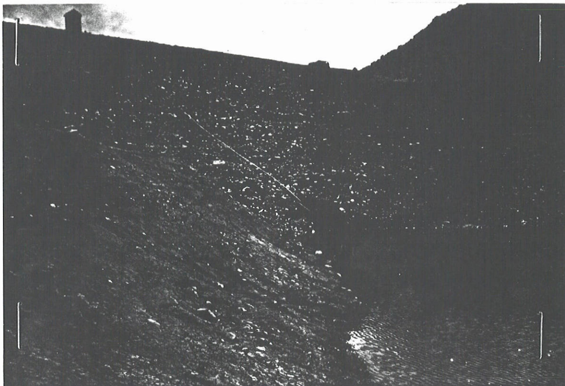
Looking South west at the control gate
