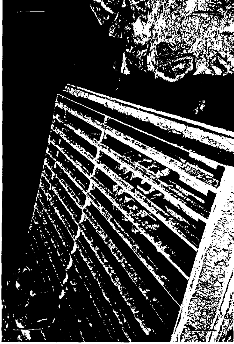
Facing looking North and down looking down at the control gate
