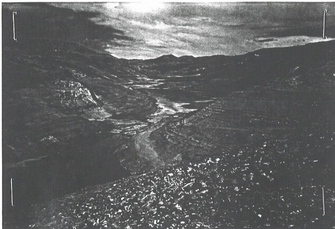
Looking Nor- east at the reservoir area from the top and center of the dam.
