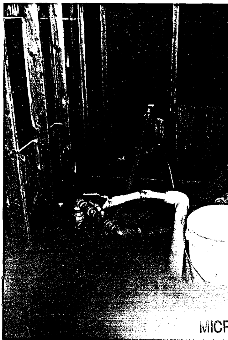
PICTURE # 2. SHOWS INSIDE OF WELL HOUSE.
