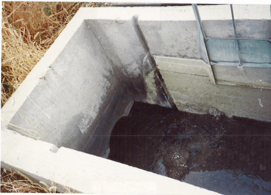
2-way concrete irrigation box - delivers to 2 12" cement culverts.
