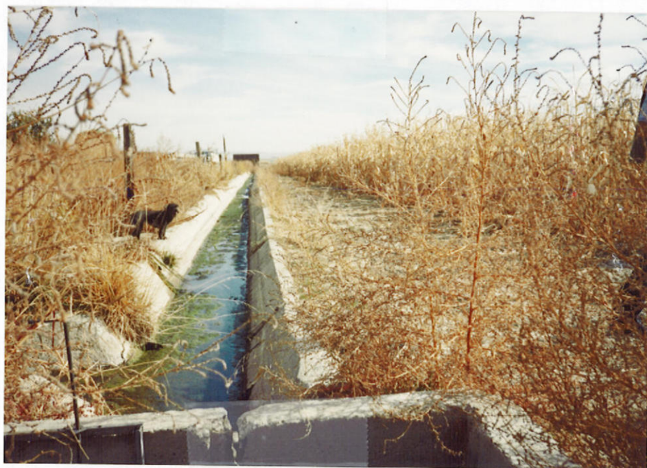
Cement Ditch where Mannings was done.
