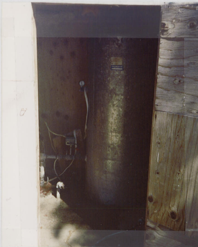
Well with power line to 3/4 hp submersible pump and discharge line to pressure tank supply, single family house, lawn, garden and stockwatering tanks.
