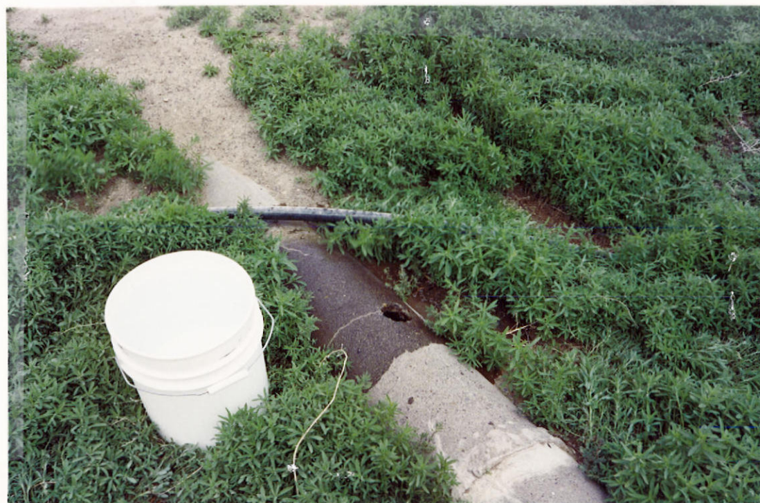
Cement ditch to which water is delivered. The artesian water is mixed with water from Oakline Irr. District.
