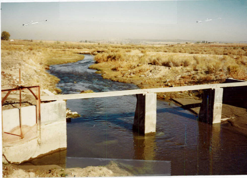
JUMP CK. DIVER- SION LOOKING DOWN- STREAM FACING (NORTH) WITH HEADGATE ON LEFT SIDE OF PHOTO.
