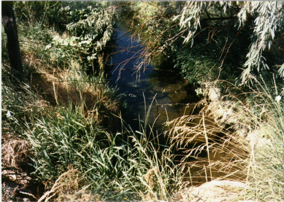
Conveyance ditch from creek, & culvert.
