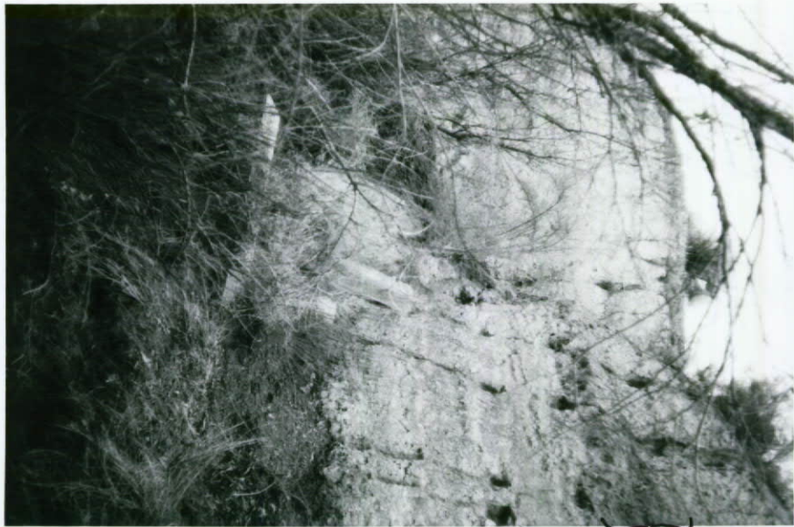
POSSIBLE HIGH WATER MARKS
