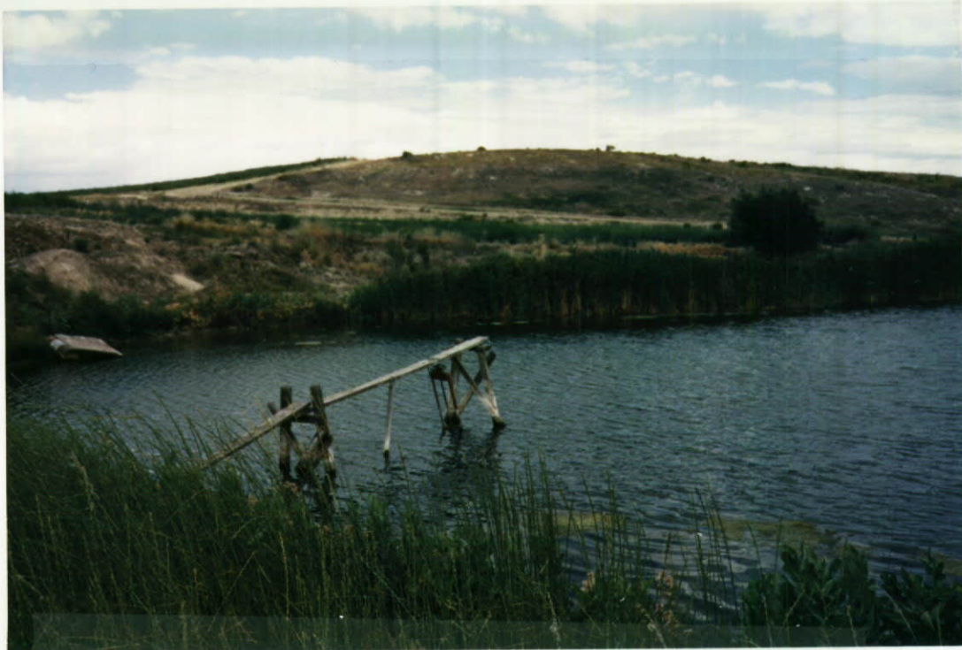
A57-00004 IS DELIVERED VIA A SCREW TYPE GATE VALVE ON AN UNDETERMINED STYLE CULVERT INTO LATERALS AND DITCHES. GATE IS ACCESSED VIA THIS BRIDGING. THE INACCESSIBLE CULVERTING FROM THE RESERVOIR ENTERS THE UNNAMED DITCH BELOW THE DAM FROM WHICH THIS PHOTO IS TAKEN.
