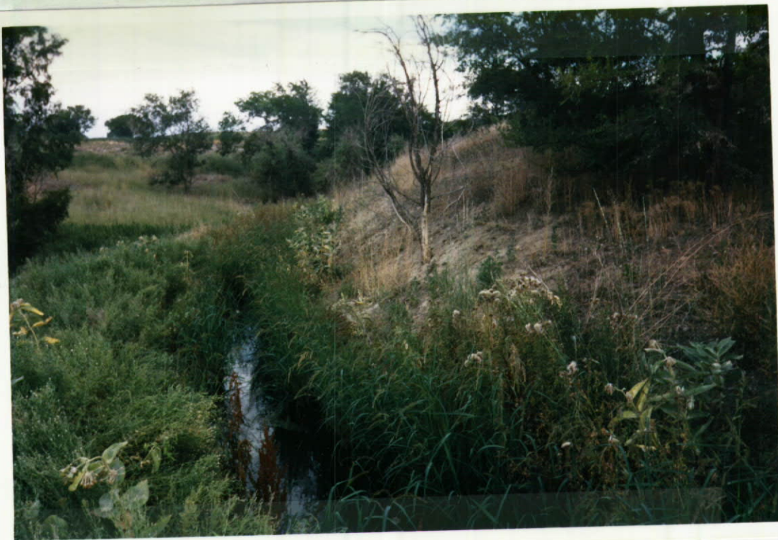
A57-00003 AND A57-00004 ARE DELIVERED VIA A SCREW TYPE GATE VALVE ON AN UNDETERMINED STYLE CULVERT INTO LATERALS AND A DITCH, PICTURED ABOVE. WATER FROM THE RESERVOIR ENTERS THE UNNAMED DITCH BELOW THE DAM AND IS THEN SPLIT TO THE TWO HALFS OF THE CONTIGUOUS FIELD DESCRIBED IN THE RIGHTS BY THE SMALLER HEADGATES AND CULVERTING PICTURED BELOW.
