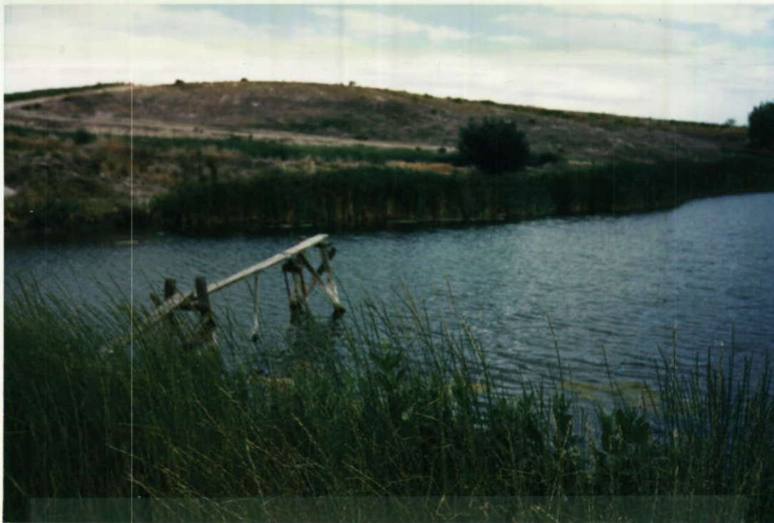
A57-00003 IS DELIVERED VIA A SCREW TYPE GATE VALVE ON AN UNDETERMINED STYLE CULVERT INTO LATERALS AND DITCEHS. GATE
