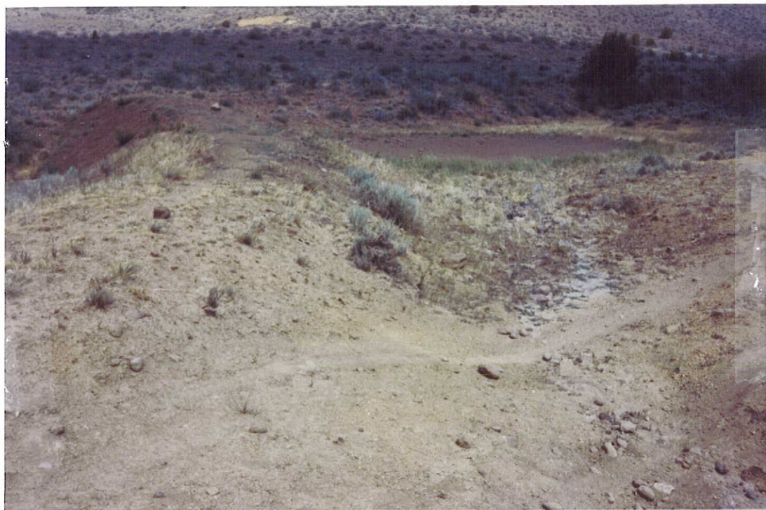
Dirt Dam & Ditch - P/D on Toppin Creek - Looking upstream towards dam.
