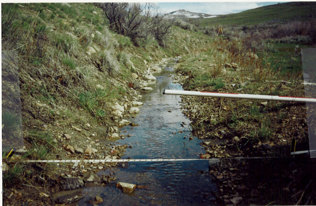
NORTH DITCH, DOWNSTREAM SECTION. LOOKING UPSTREAM TOWARDS LEVEL.
