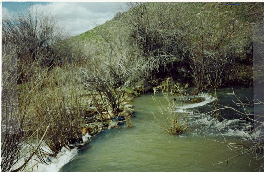
P/D #1 WOOD GATE ACROSS COW CREEK, NORTH DITCH.
