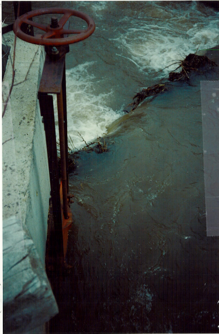
UPPER P/D OUTLET TO WEST DITCH.
