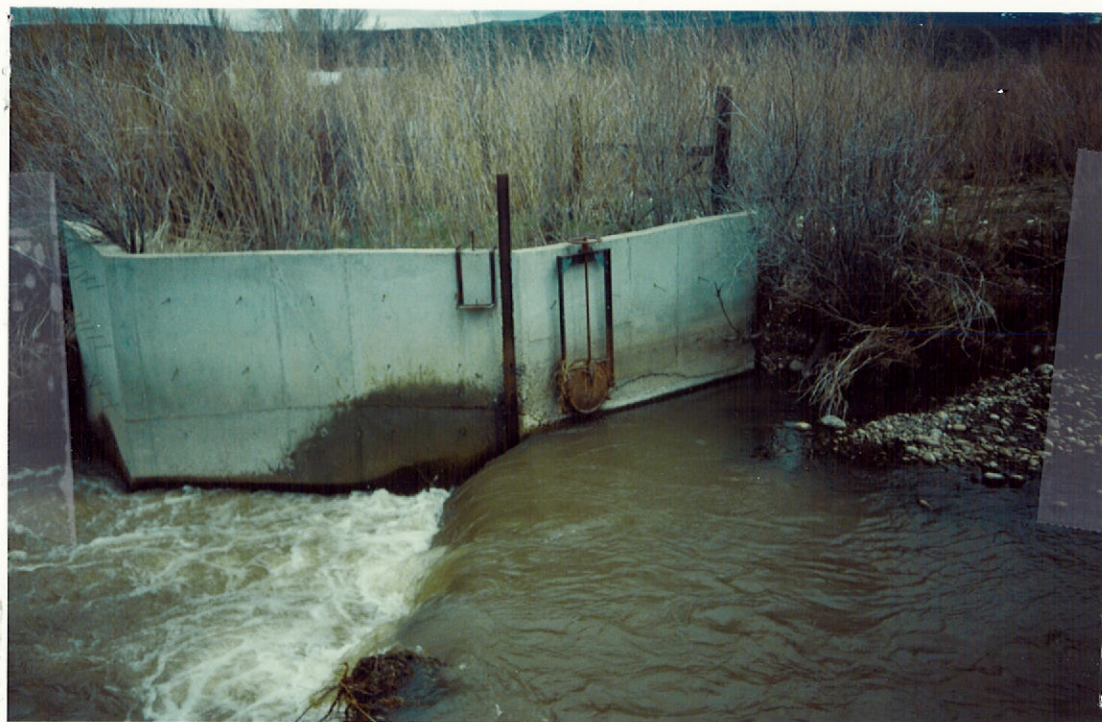
OUTLET TO EAST DITCH.
