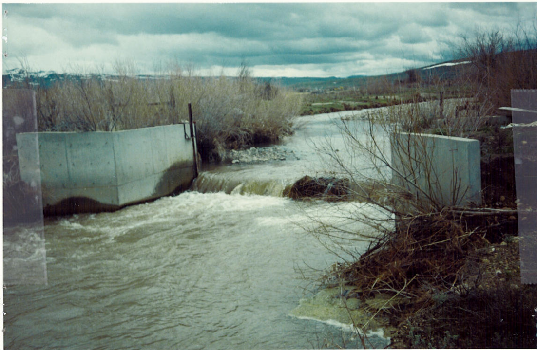
UPPER P/D (CONC. DAM) USES BOARDS IN CENTER.
