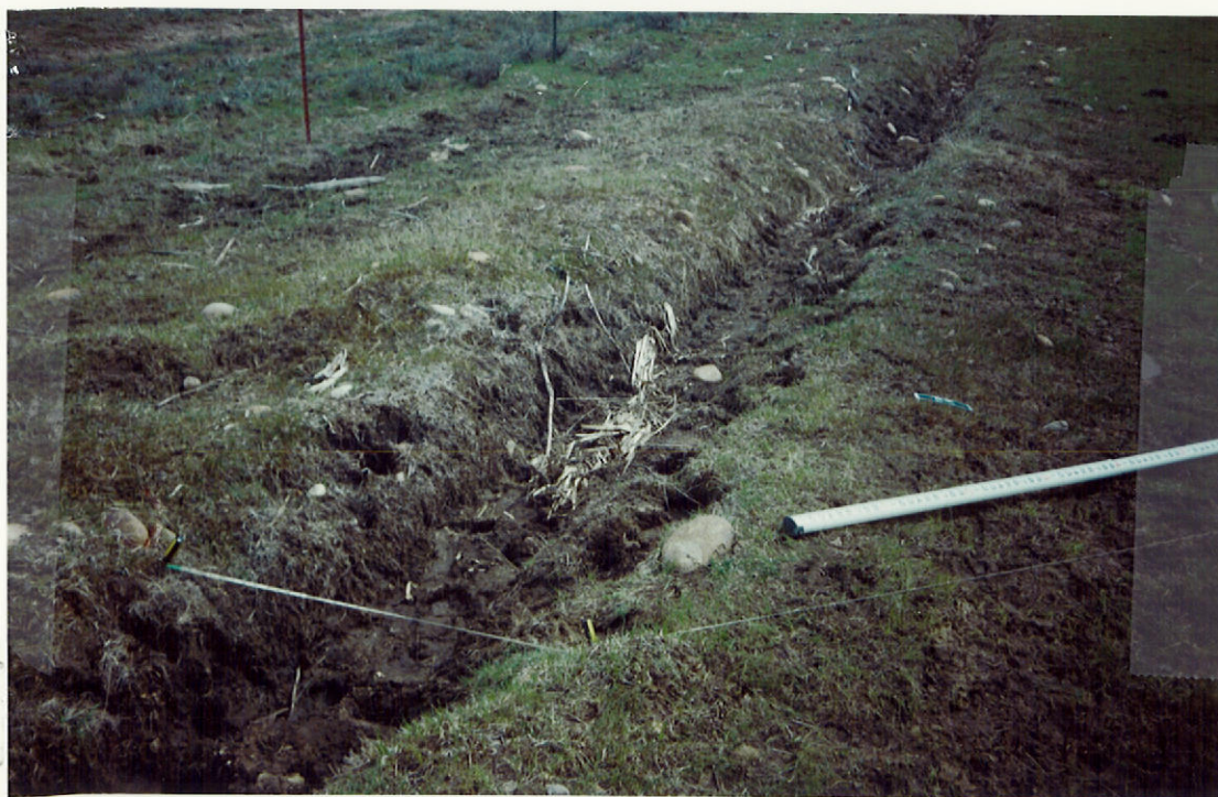
WEST DITCH, UPSTREAM SECTION, LOOKING TOWARDS P/D.
