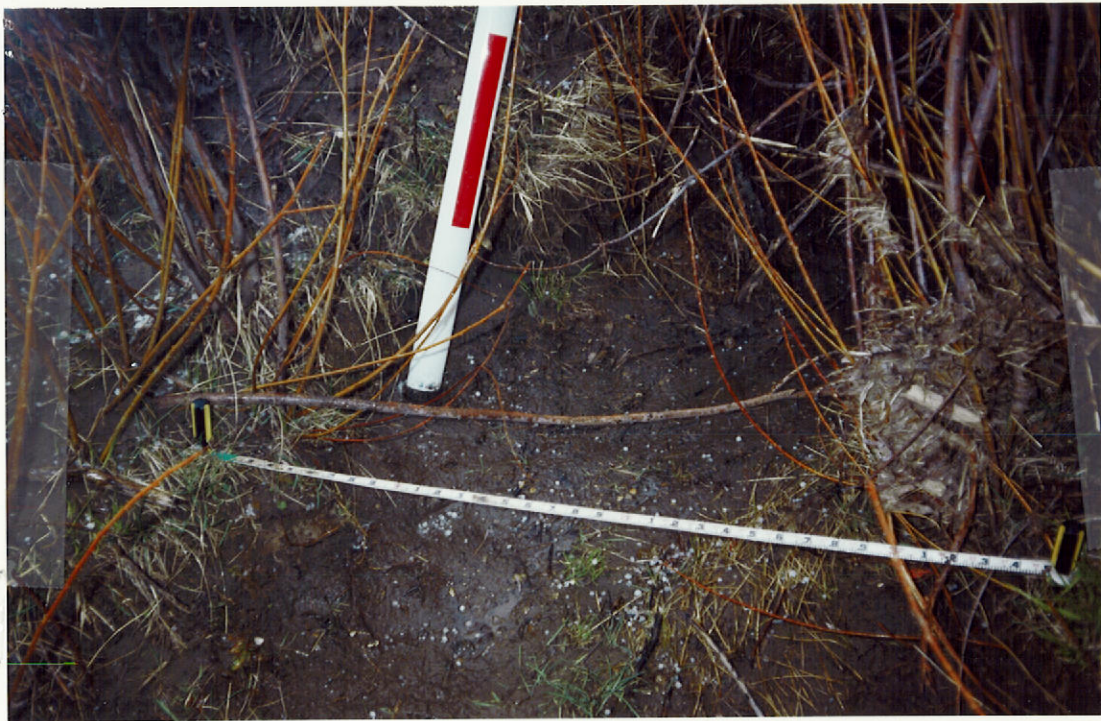
EAST DITCH, UPSTREAM X-SECTION, TOWARDS P/D.
